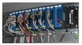
When you face problems with Compact Field Point I/O electronic modules from National Instruments (I/O CFP hereafter), the following FAQ could help.
