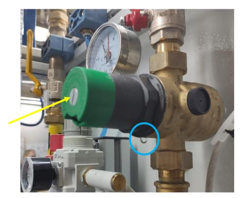
Water leak, blue circled in the picture, is usually fixed by tightening the screw located in the middle of the front green knob (see yellow arrow).
